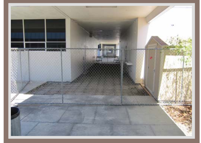
Newark Jr. High School Concrete Replacement
