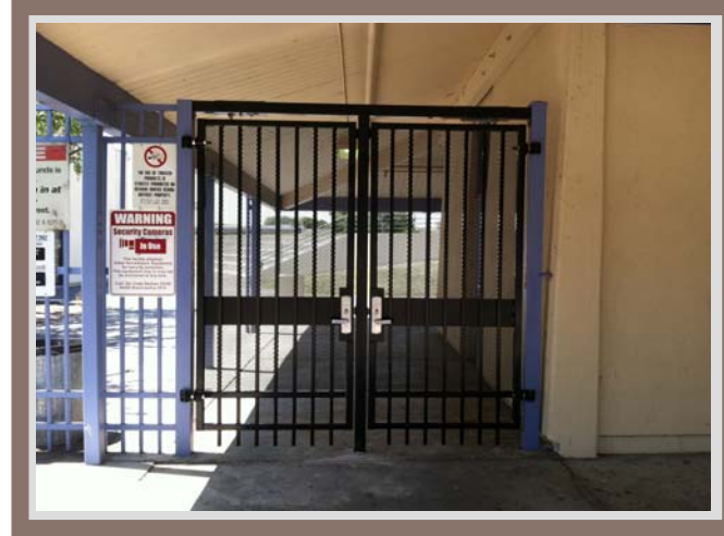
NMHS Gate Replacements and Panic Hardware
