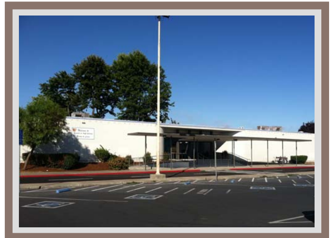
Newark Jr. High School Entry Upgrade
